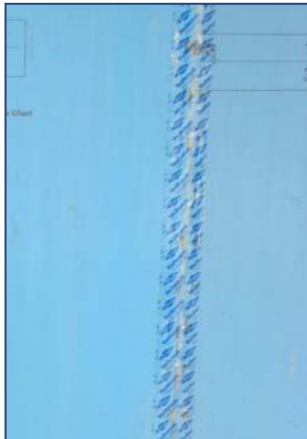
4) If foam sheathing will function as WRB, tape seams according to manufacturer's instructions.
