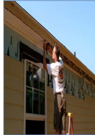
6) Install siding according to manufacturer's instructions.
