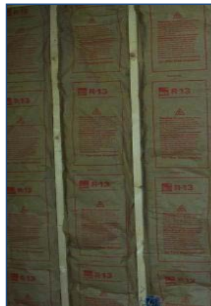
4) Insulate 2x4 wall.
