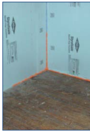
2) Install rigid foam and air seal.
