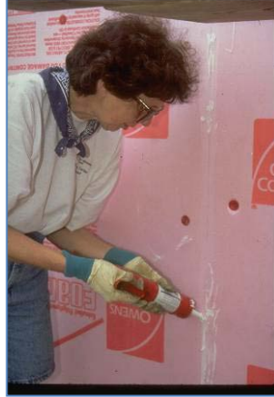
2) Secure insulation using plastic cap nails.
