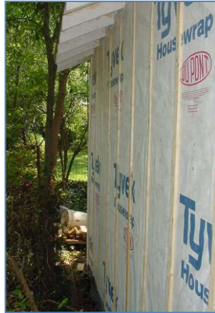
5) If siding is installed in a rain screen configuration install furring strips attached directly to the underlying framing.
