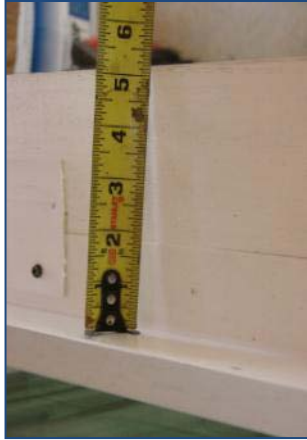
1) Extend door and window jambs as necessary.
