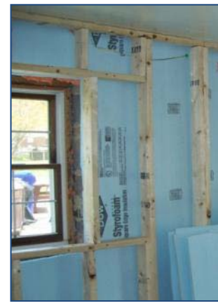
3) Construct 2x4 wall.
