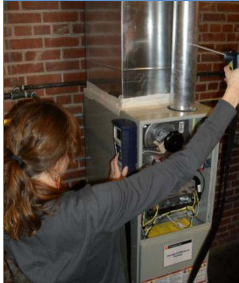
Figure 4. Draft Pressure Testing using Combustion Analyzer.
