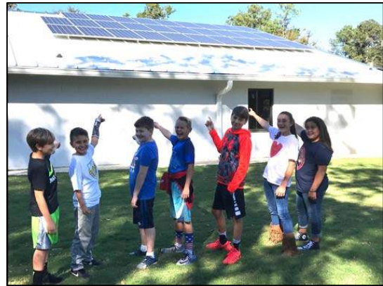
The Chatsworth Club's 9.8 kW solar system was installed in February 2017.
