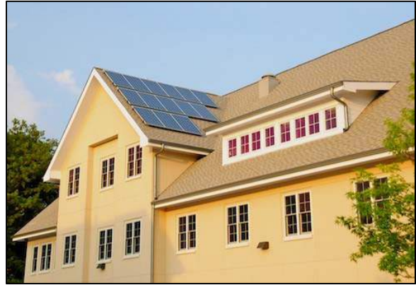
Chris Kids installed a 23.7 kW system in 2011 via funding from the Georgia Environmental Finance Authority.
