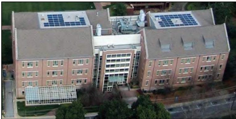
Bullock Science Center - Agnes Scott's first solar array, which was installed in 2013 as part of Georgia Power's ASI.
