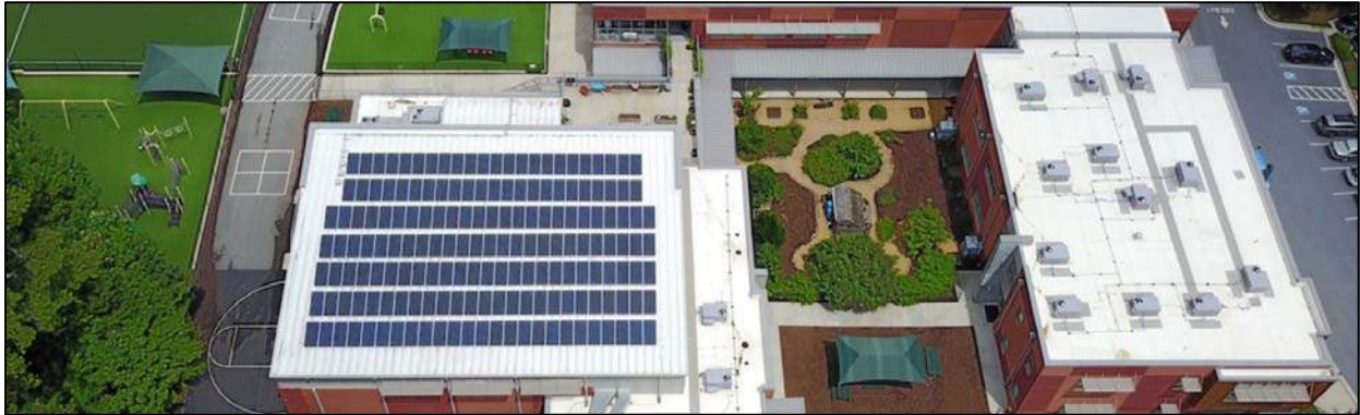
Cliff Valley School's 59 kW system is installed on the roof of its gymnasium.
